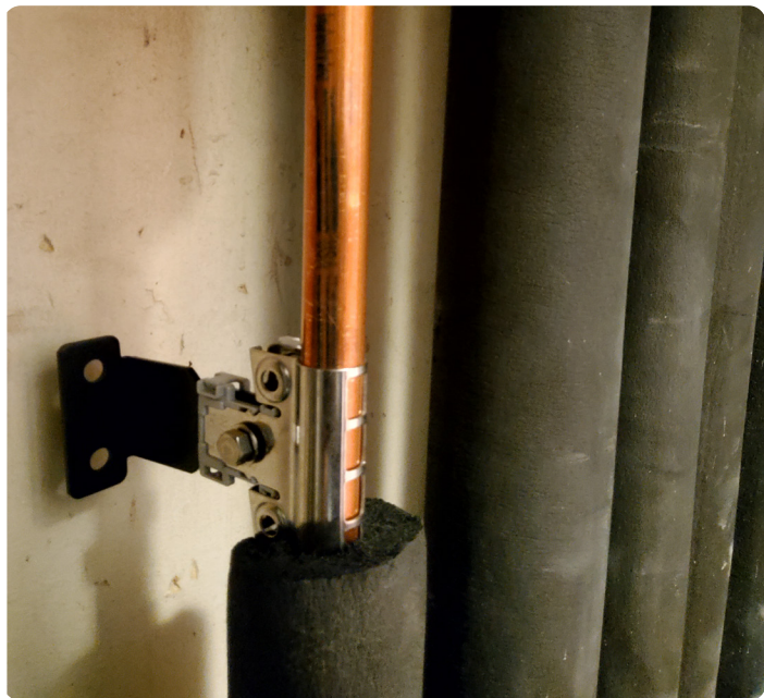
LineBrace being installed in the shaftway.
