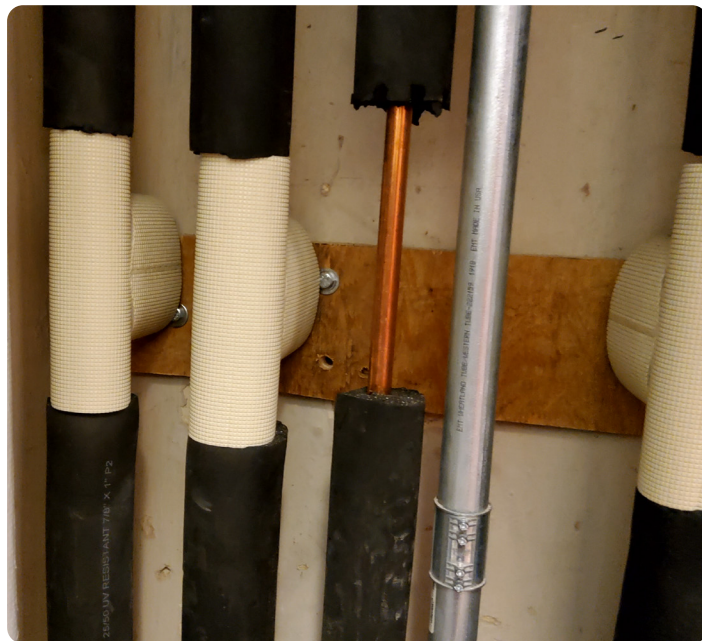
LineBrace installed and covered by the thermal sleeve.
