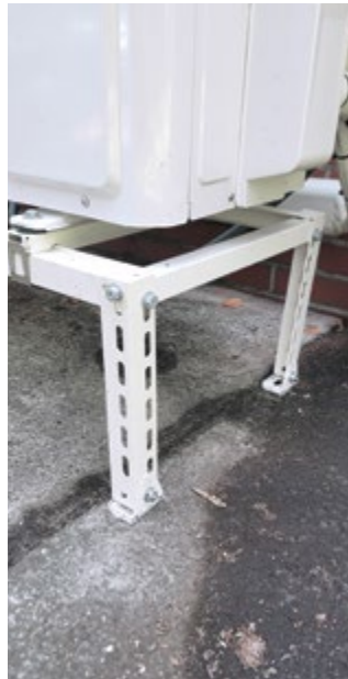
Paircoil and Slimduct SD going into the condenser with C-NG-L slab support.
