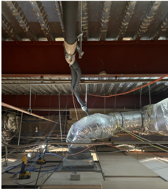
SuperLock holding the refrigeration pipe.
