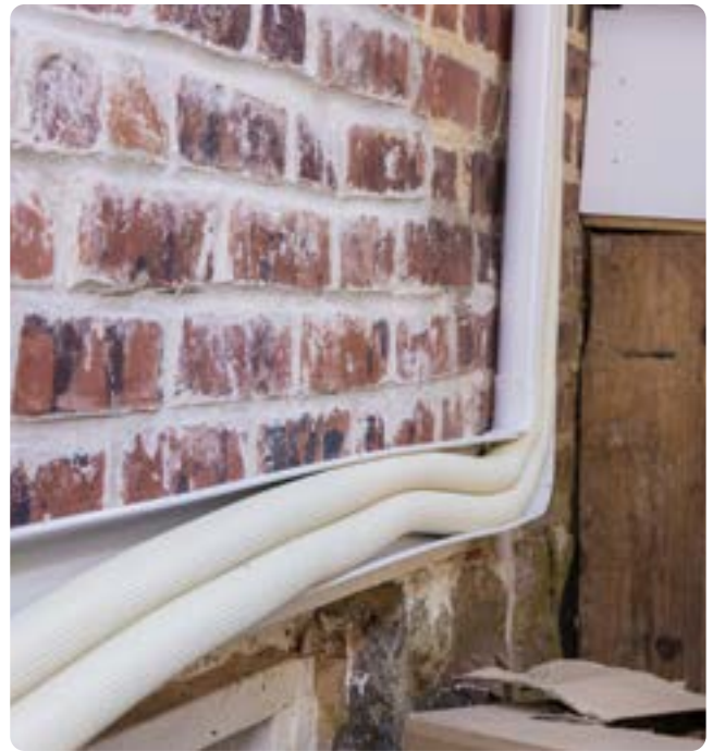
Paircoil lineset inside Slimduct SD lineset cover 77 Ivory.
