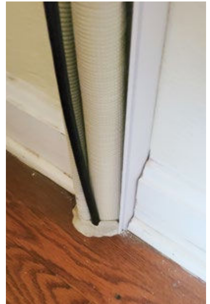
DHQ drain hose and Paircoil inside Slimduct MD sealed with AP Putty in the closet.
